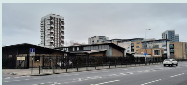
Figure 10. Images showing current conditions at Site 1
